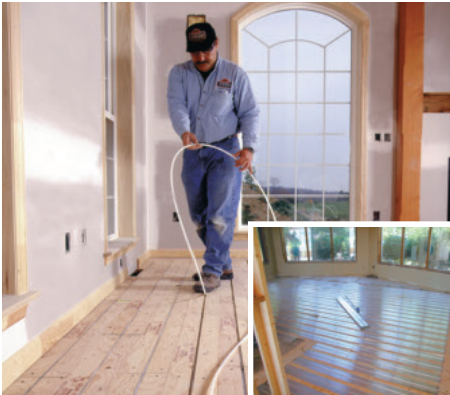
Low mass dry system option - thin profiles simplify basement and above subfloor retrofits.
