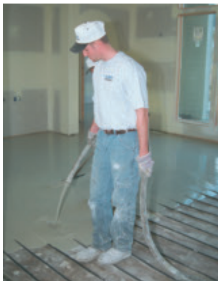
Material costs are typically lower for over-pour systems when compared to low mass systems
