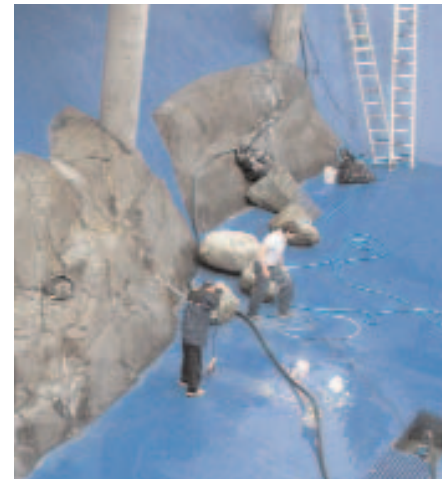
Waterscape construction underway at Vancouver Aquarium Marine Science Centre.
